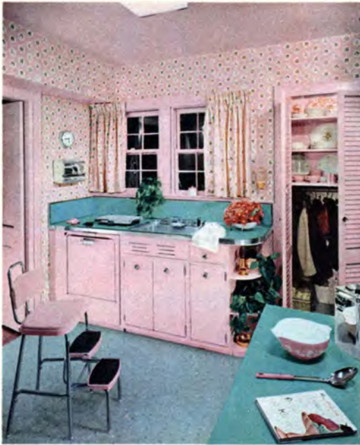
No structural changes were made in remodeling. New sink was placed a few inches to the right of the old one to make room for dishwasher that stood in closet. Only minor plumbing changes were needed
